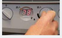
Turn the knob clockwise to increase or anticlockwise to decrease the temperature. Range 25 - 80°C.
